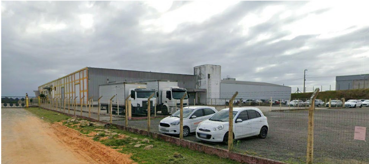
Minamel Agroindustria Ltda's ("Minamel") honey processing facility (courtesy of Google EarthPro)
